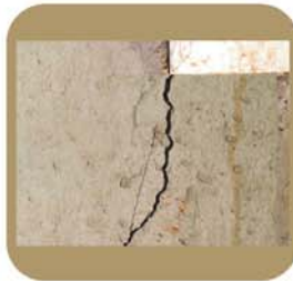
Foundation Crack
